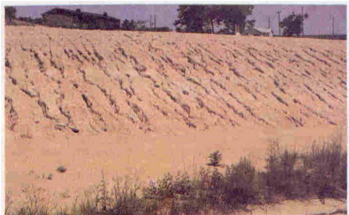
Erosion in Slopes
